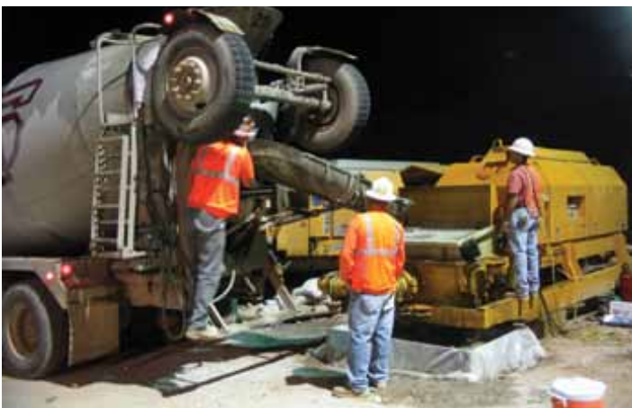
Fig. 4: Concrete truck discharging into the concrete pump (photo courtesy of Obayashi/PSM JV)
