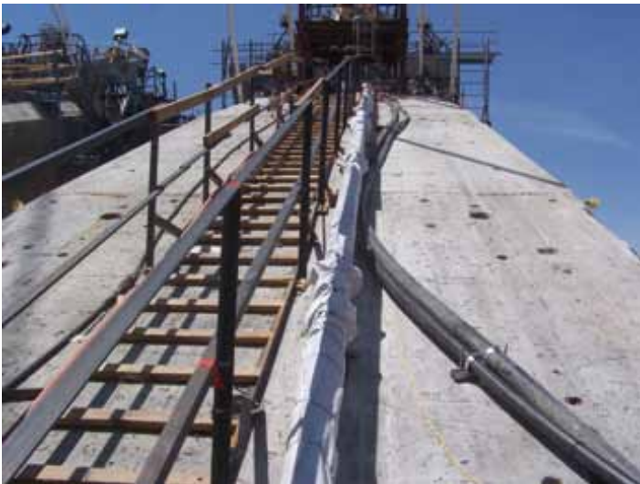
Fig. 3: The concrete slickline wrapped in burlap. Soaker hoses inside the burlap delivered chilled water to the exterior of the slickline in an effort to reduce concrete heat gain during pumping (photo courtesy of Obayashi/PSM JV)
