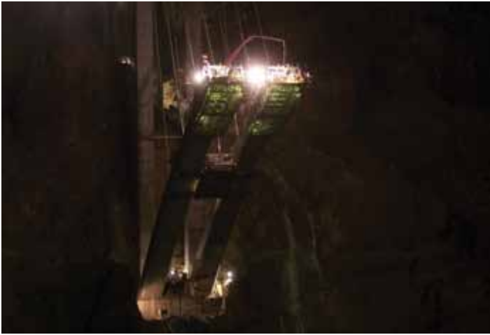
Fig. 8: A typical night-time concrete placement on the arches using the placing boom (photo courtesy of Obayashi/PSM JV)
