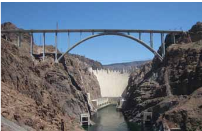
Fig. 9: An overview of the nearly completed bridge on August 20, 2010 (photo courtesy of Obayashi/PSM JV)
