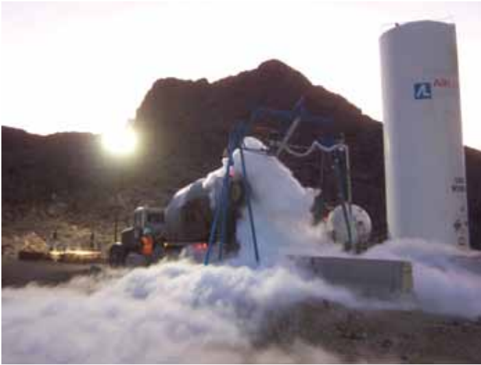
Fig. 2: Liquid nitrogen being injected into a concrete truck (photo courtesy of Obayashi/PSM JV)
